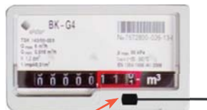
Built-in magnet in the gas meter
